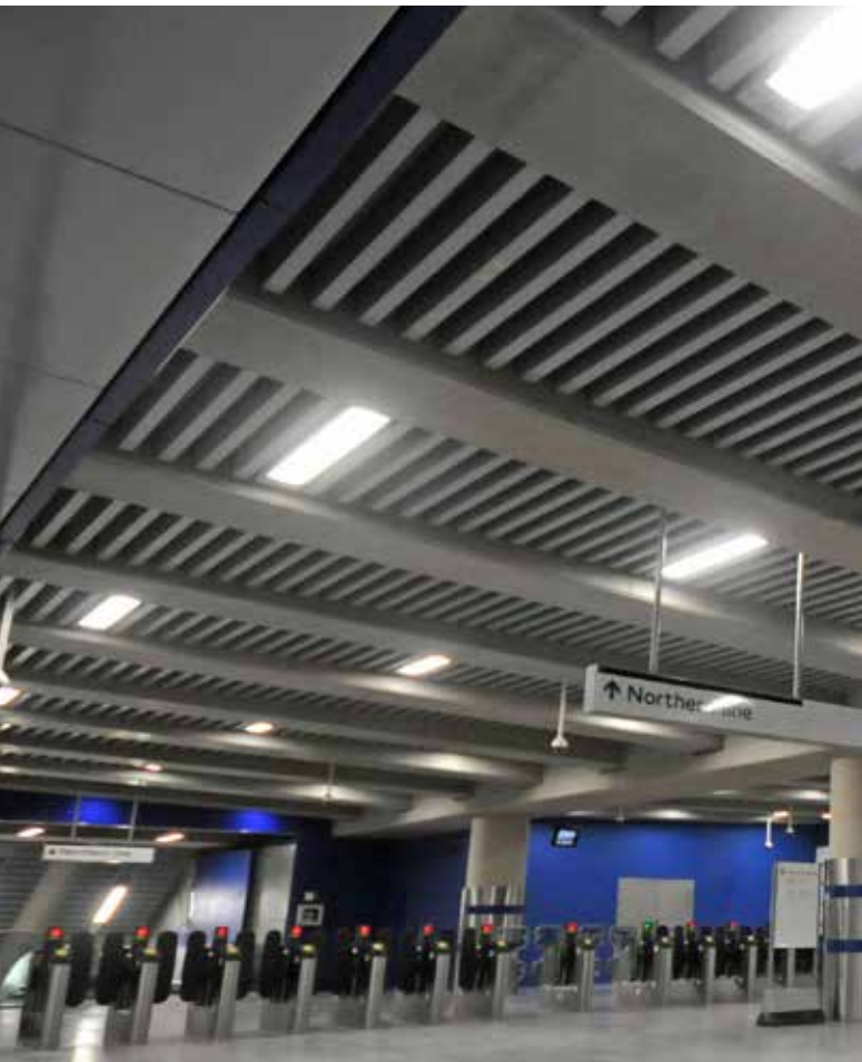
Tottenham Court Road, London: Bespoke baffles
