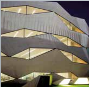
2010 - Vodafone Oporto Portugal (Completed)
