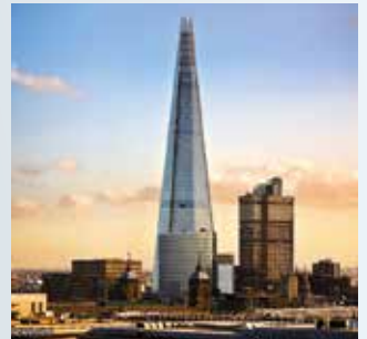
2012 - The Shard (Completed)
