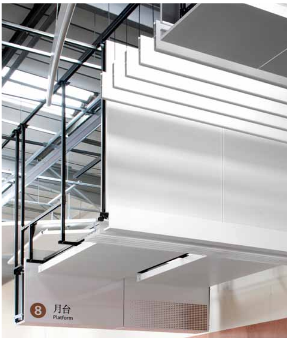
Train platform bespoke ceiling system consisting of 2mm thick aluminium fabricated operable panels, decorative straight and curved baffle extrusion 300 x 50 x 3mm.
