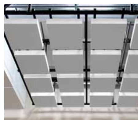
Project ceiling system type 4 a nominal 1500 x 1500 module consisting of a 600 x 600 x 2mm fabricated aluminium operable tile.
