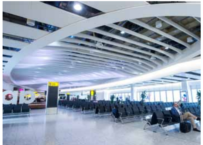
Heathrow Airport, Terminal 4 Acoustic baffles
