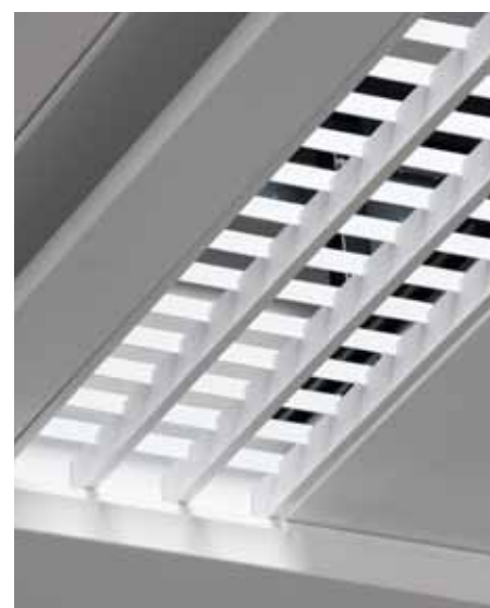
Project ceiling system type 3 a nominal 1500 x 1400 module consisting of a 800 x 900 x 2mm aluminium operable tile. Running parallel either side of the panels are continuous lengths of decorative grilles.
