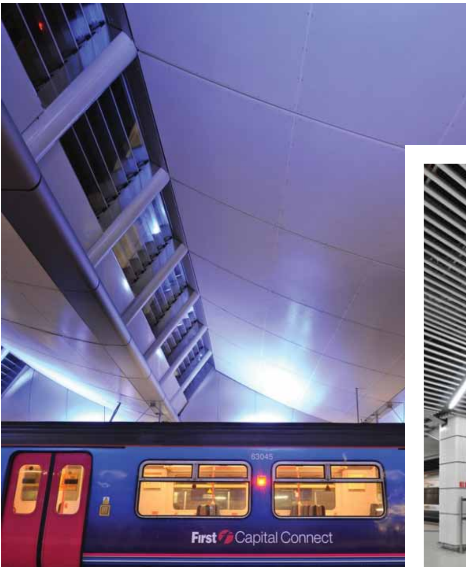
Blackfriars Bridge Station, London Bespoke soffit lining with triangular metal panels
