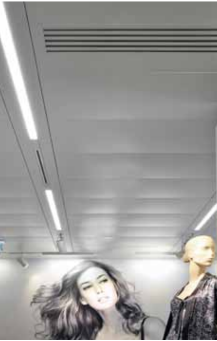
Marks & Spencer, So Ouest, Paris System 330 ceilings
