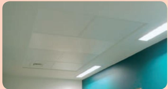
Radiant heating systems are easy to access and their flat surfaces are easy to clean. Current deep clean guidance requires the removal of traditional radiator covers and cleaning behind radiators which can be both difficult and time consuming.
