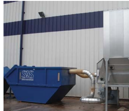
Wood dust extractor
